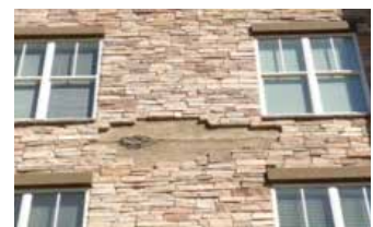
Adhesion Failures
